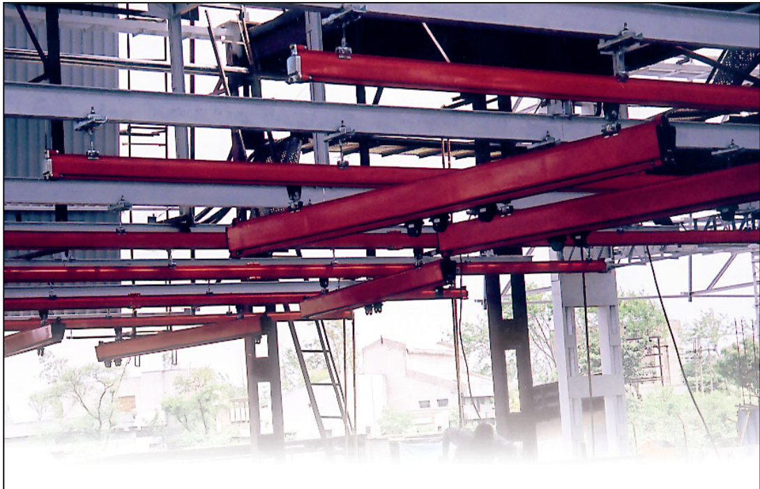
BF Gantry System Installation at HCV Plant
